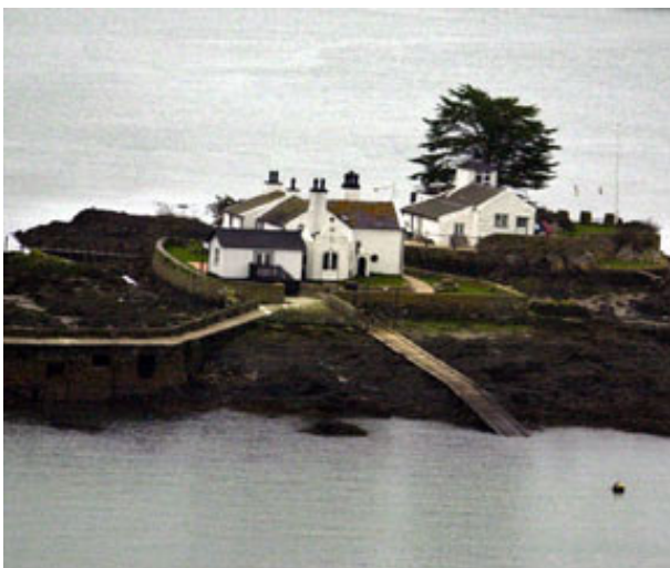
Figure 1. Land restrictions at buildings near the sea afford an opportunity for mooring a small wind turbine just a short distance offshore and supplying power back to the building via marine cable.
